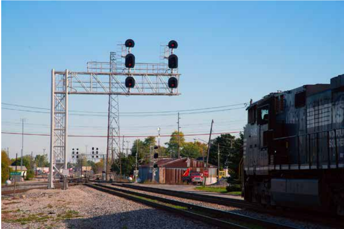
Bellevue Ohio approach from the south, as seen from Kemper Rail Park.
